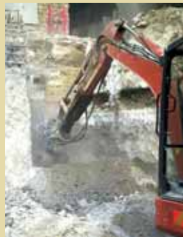
Building renovation and demolition
