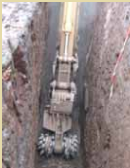
Trench and pipeline construction
